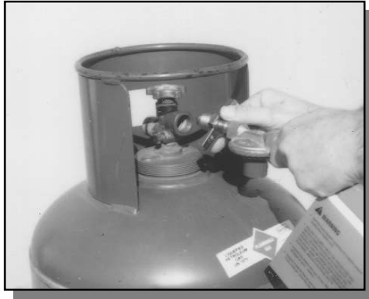
Regulator With Vent Pointing Down
